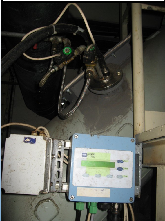
HK2 pin antennas with cleaning function Sugar
